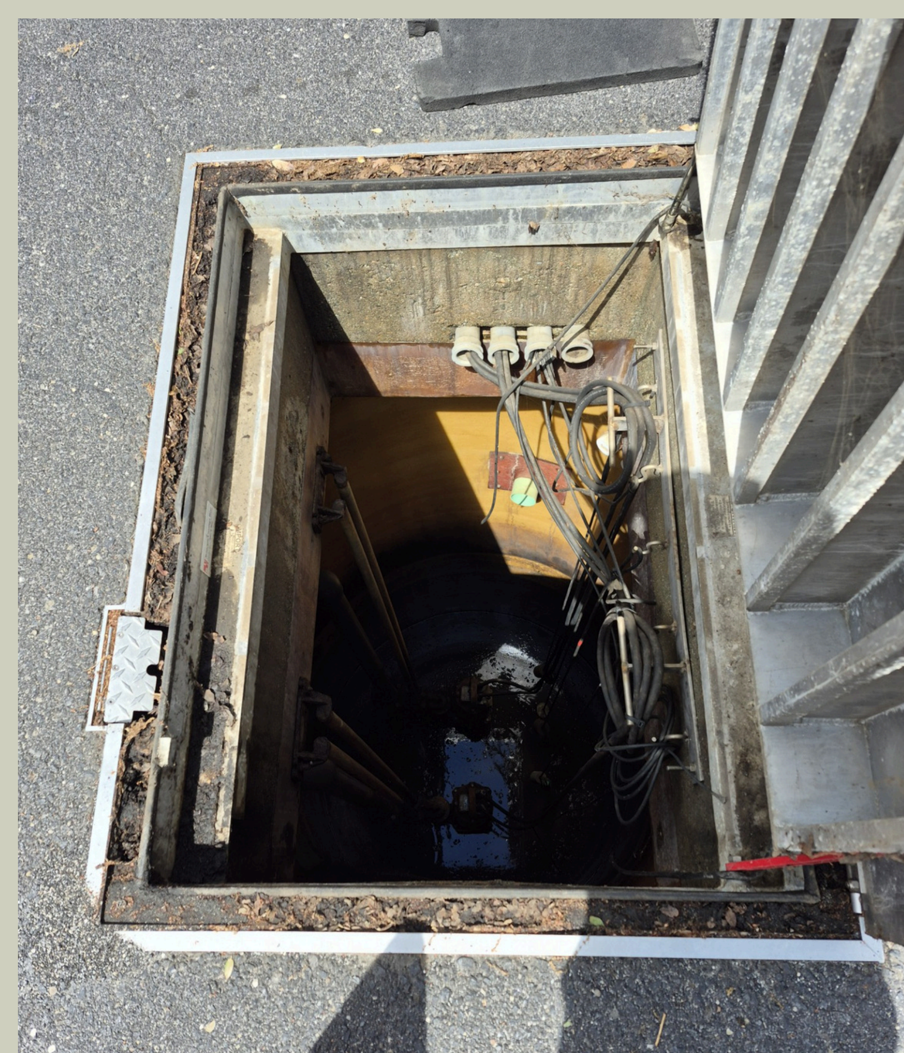
Lift Station 11 in backup - found floats failed - Poker Flat
