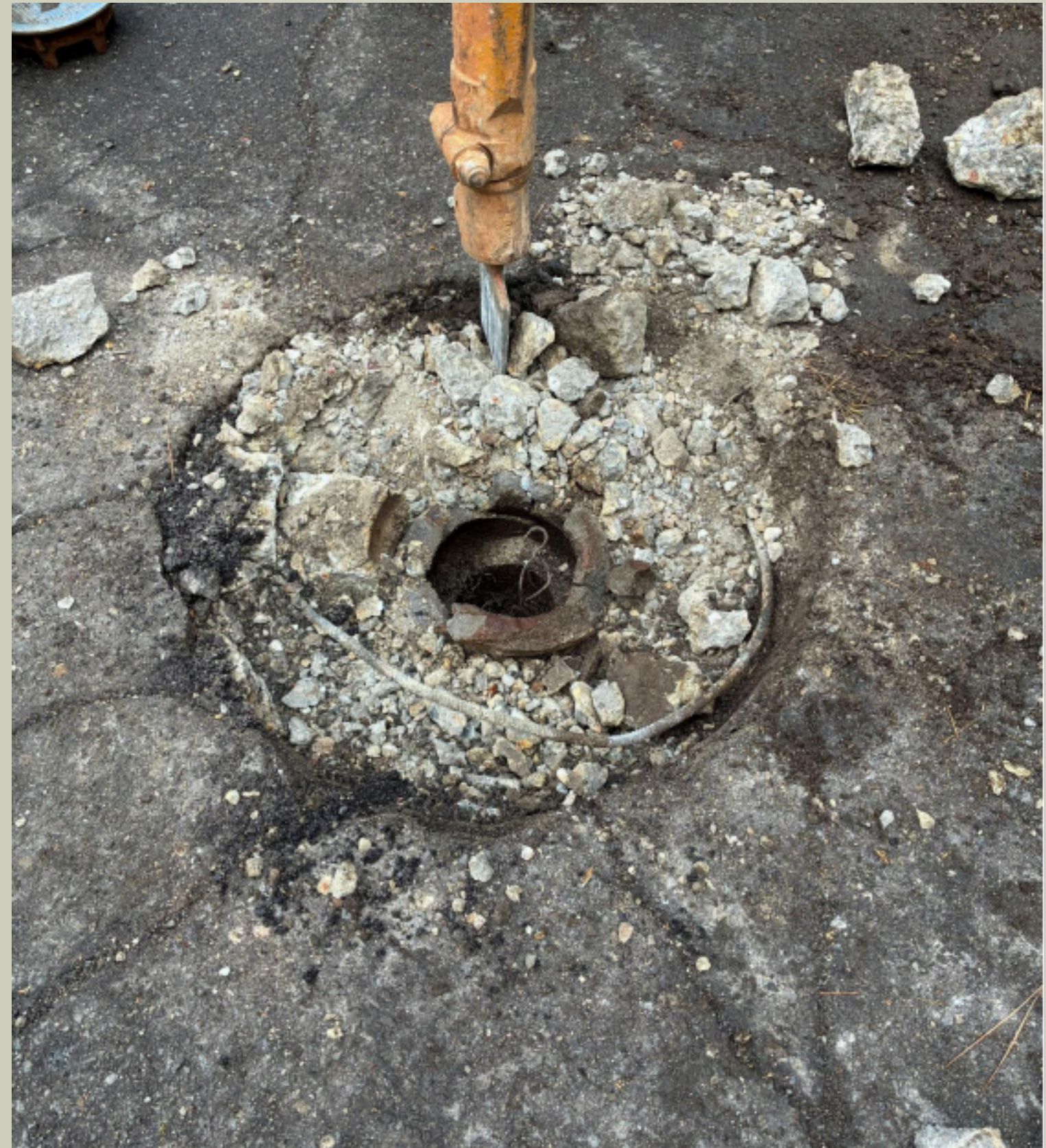
Foster Court - Reset 3 G-5's & Repaired Broken G-5 Lakewood - Ebbett's Pass
