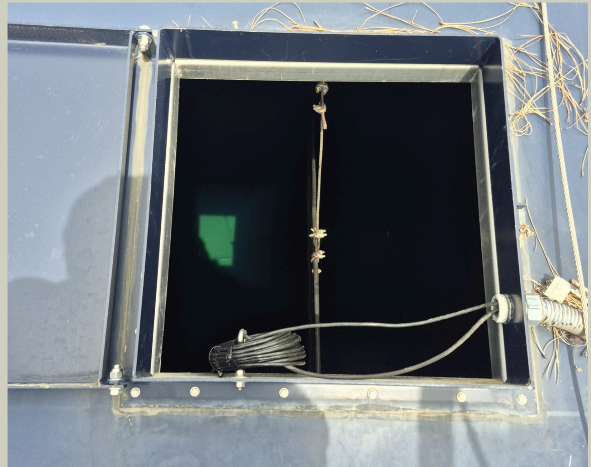
Troubleshoot and repaired Clearwell level issues - West Point WTP
