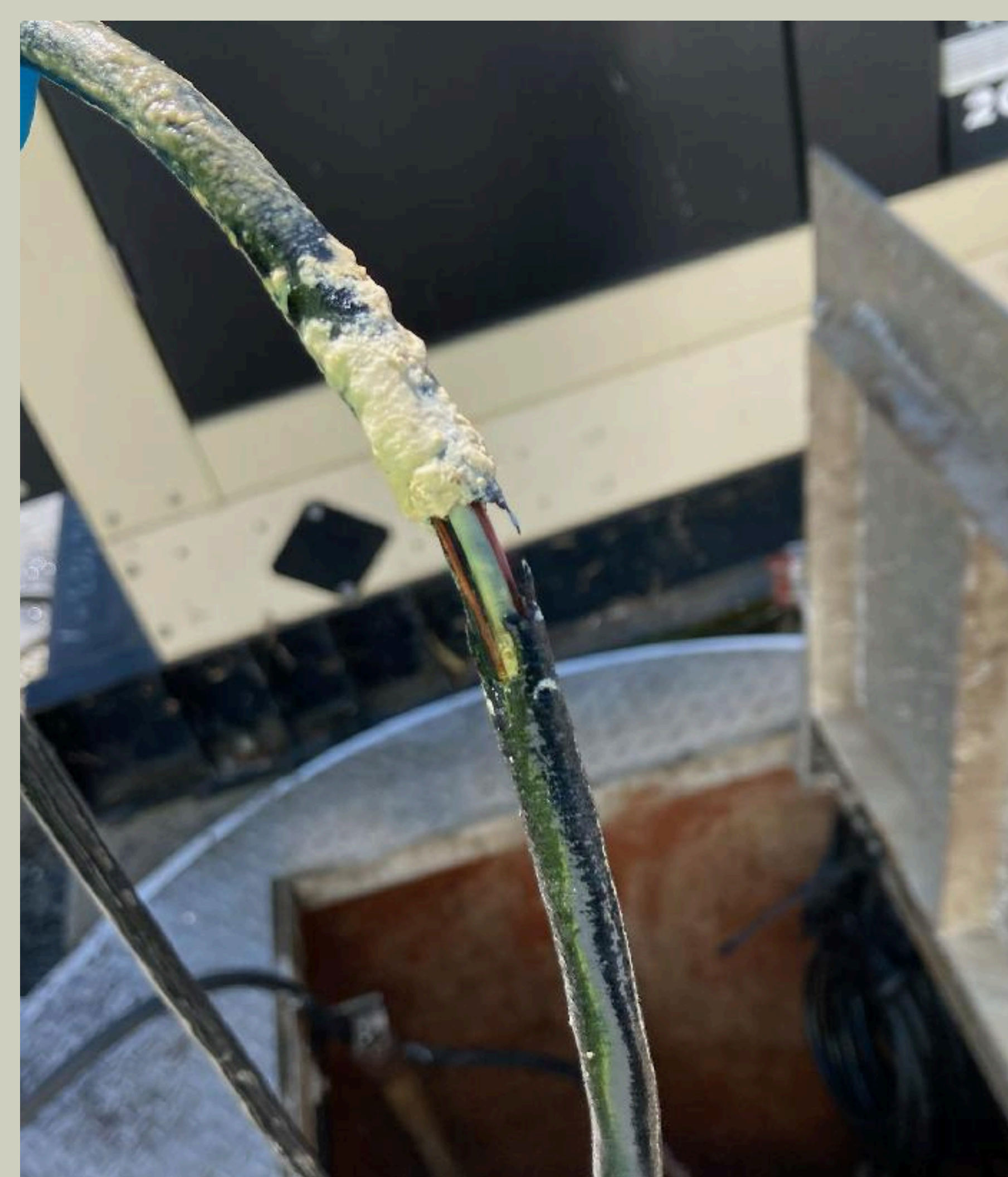
Replaced a failed float at LS 4 - Copper Cove
