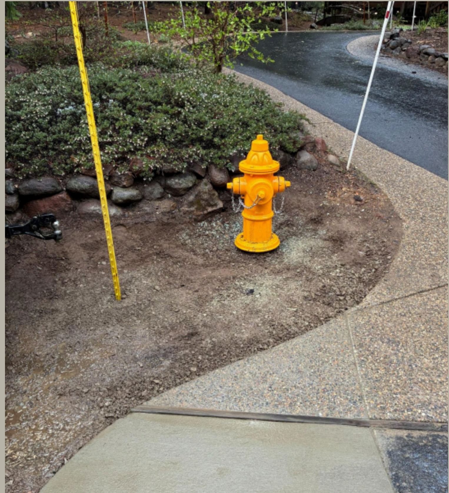
Navajo & Apache - New tee, inline valve, hydrant, & site work - Ebbetts Pass
