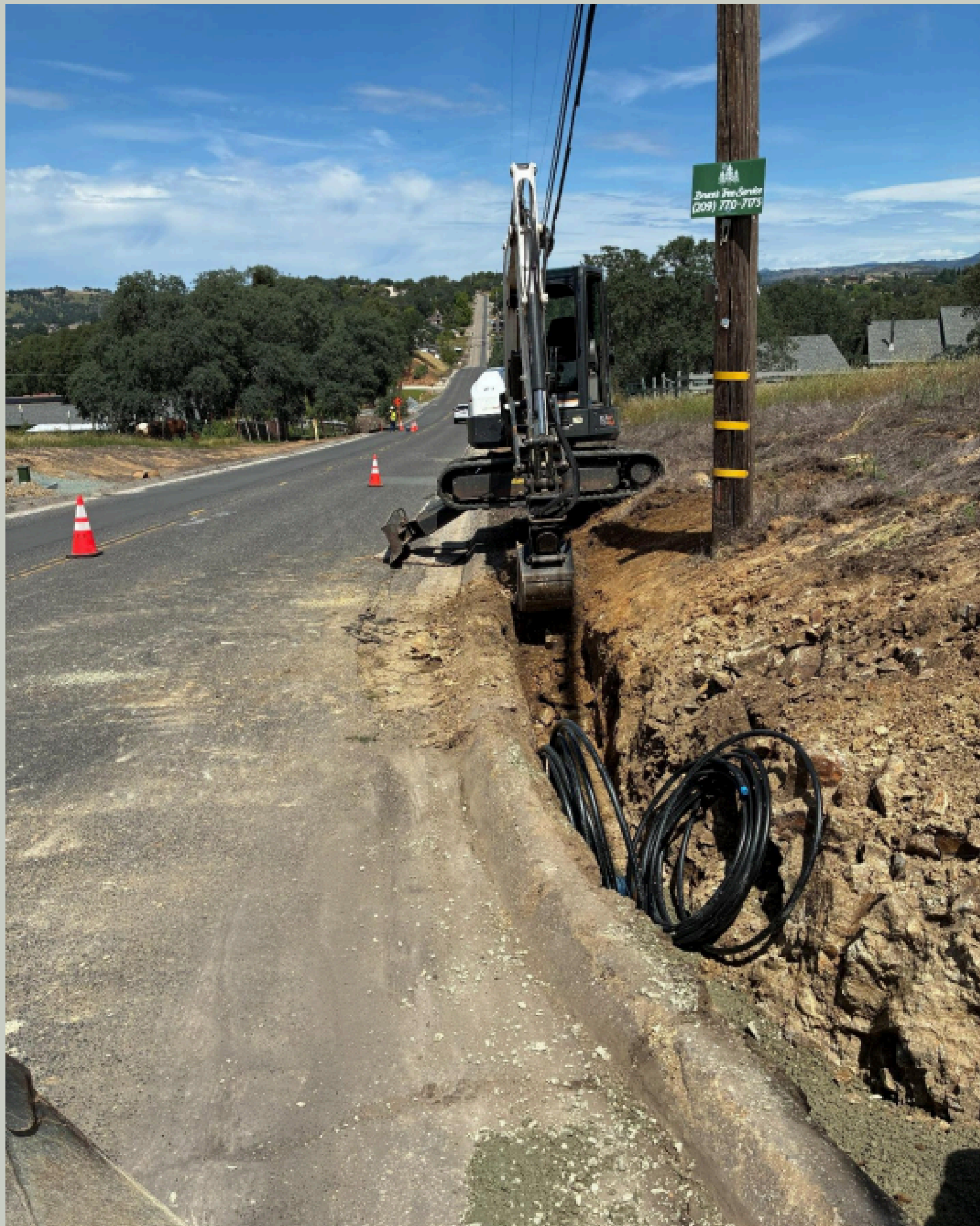
Service Line installations on 12-inch main - Dunn Rd- Jenny Lind
