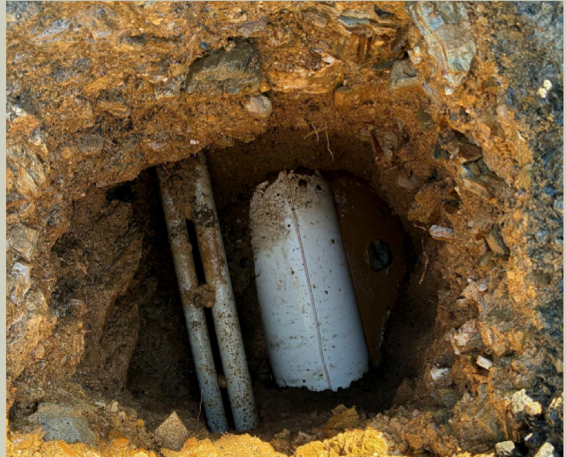
Potholing for the SAF Unit Install - Copper Cove Reclaim
