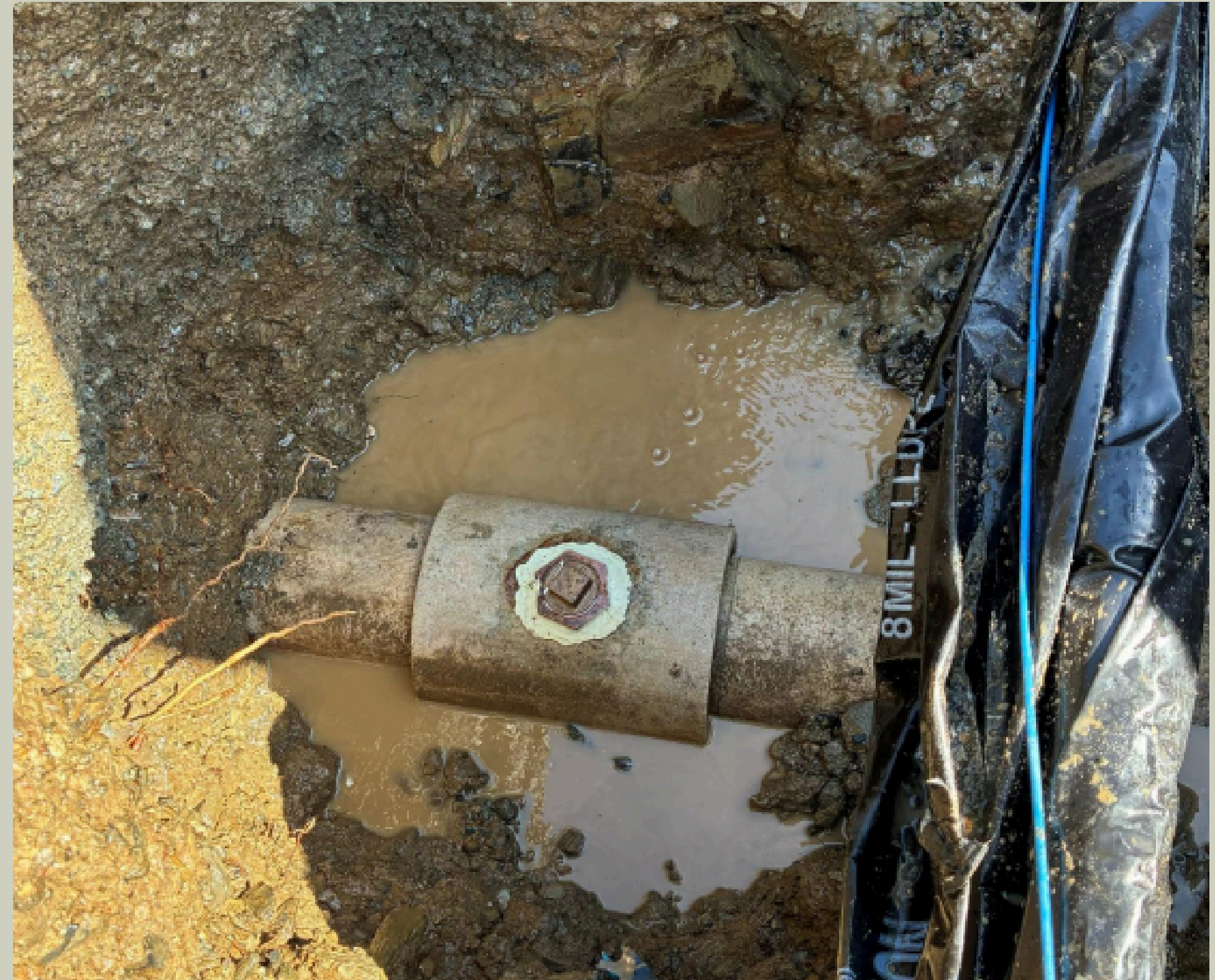
Eliminating an old blow-off - Little John Rd. Copperopolis
