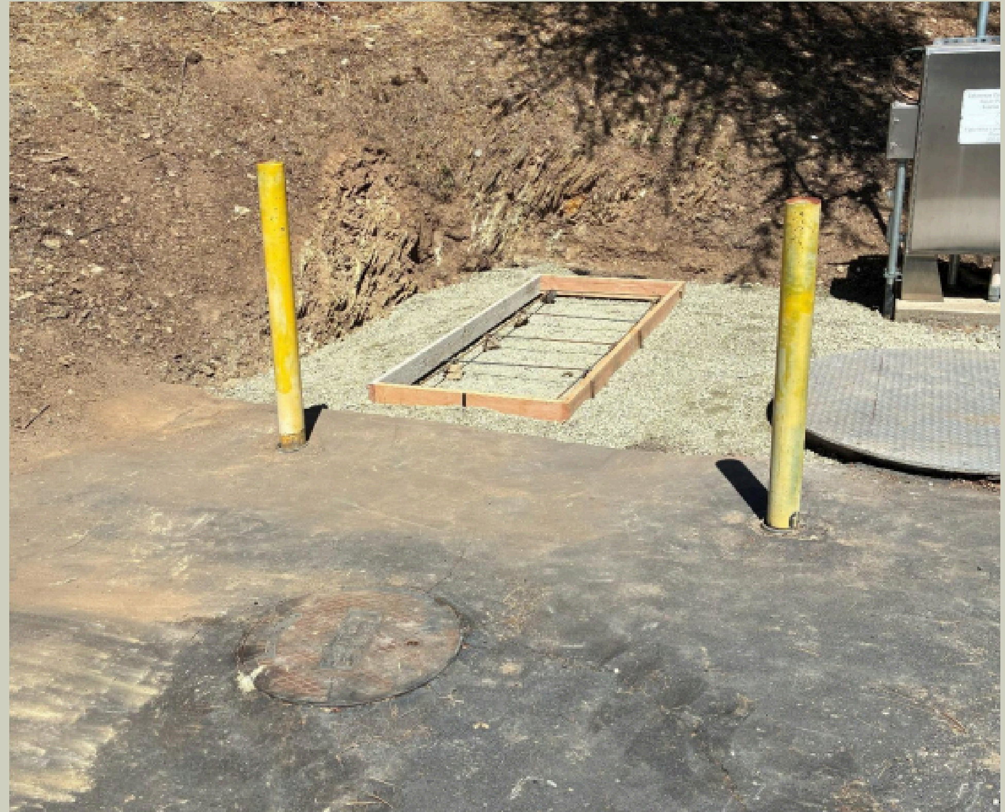
Critical Facility Generator Project - Copperopolis
