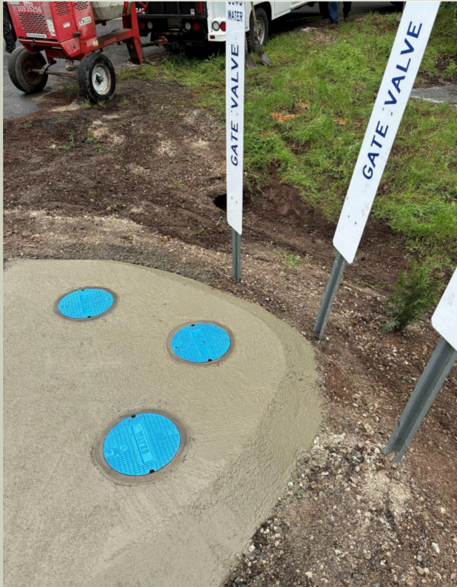
Foster Court - Reset 3 G-5's & Repaired Broken G-5 Lakewood - Ebbett's Pass
